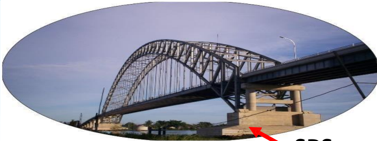
The base of the bridge SPS
