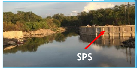
Retaining The River Wall
