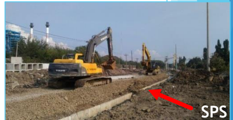
The base of the railway
